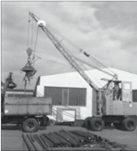
1962: rope-driven S833 with elevated operator cab
